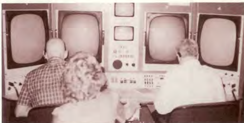
The control console of a modern T-38 flight simulator is a far cry from the old plotting table. Operators can provide any type of instrument approach or malfunction and really monitor the student's performance. IFC uses the simulators to evaluate procedures and approaches for validity, applicability, and safety.
