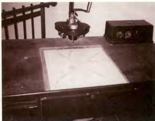
While the pilot flew the trainer through various climbs, turns, and descents, his course was traced in ink on the map on the table. After the flight, the instructor and the pilot could review the lines on the map to determine what the pilot had done.
